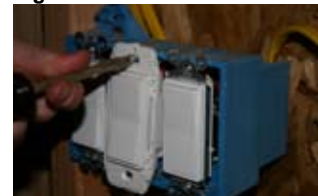
Figure C: Switch Box Mount
