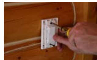
Figure C: Switch Box Mount
